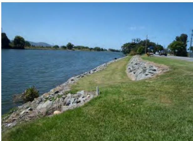
Figure 46: Left: Recent rock revetment along Tweed Valley Way, Right: Bank erosion works incorporating habitat elements (tree logs and artificial reef-style structures)
